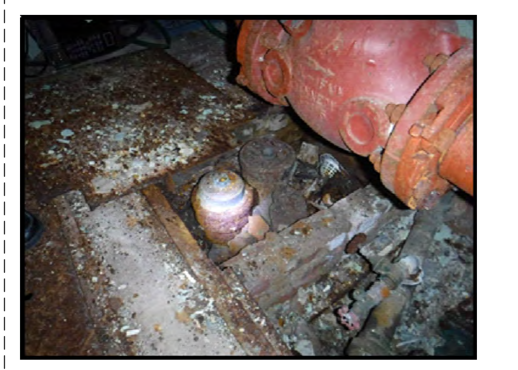
2 EXISTING HOUSE TRAP
