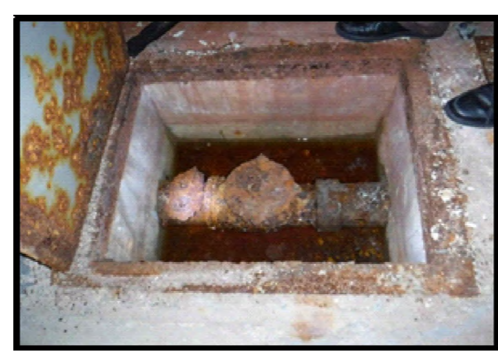
1 EXISTING BACKWATER VALVE
