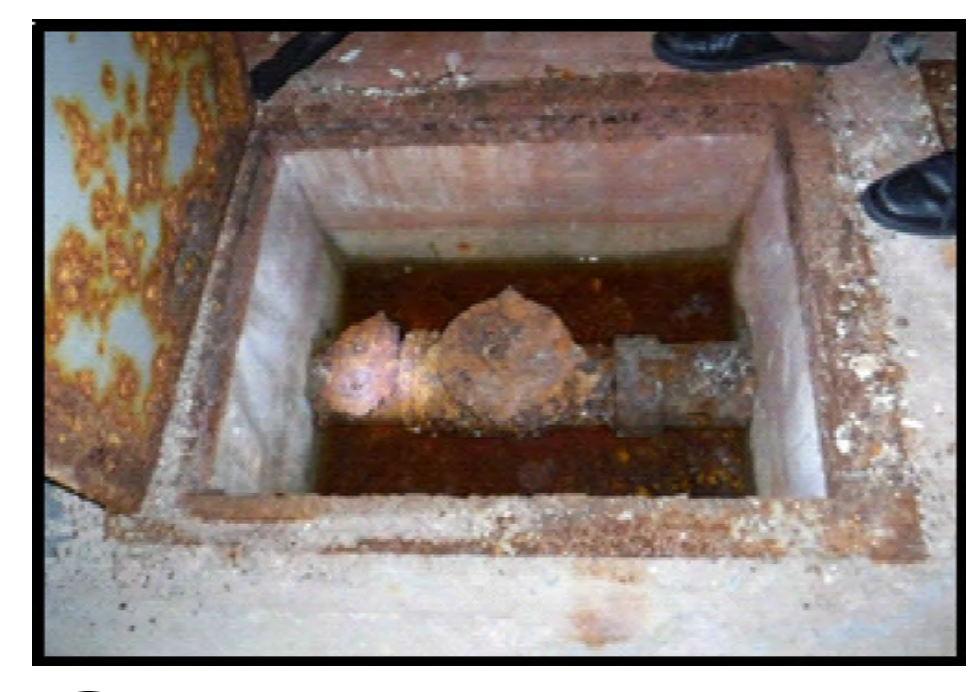
1 EXISTING BACK WATER VALVE (BWV)
